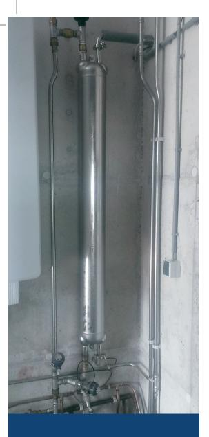
A pipe cooler cools the milk before it reaches the milk cooling tank. Heat of the milk is being removed due to cold water flowing in opposite direction of the warm milk.
